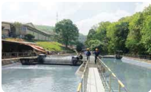
Effluent treatment plant
