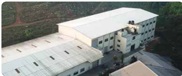
Establishment of the new knitting building
